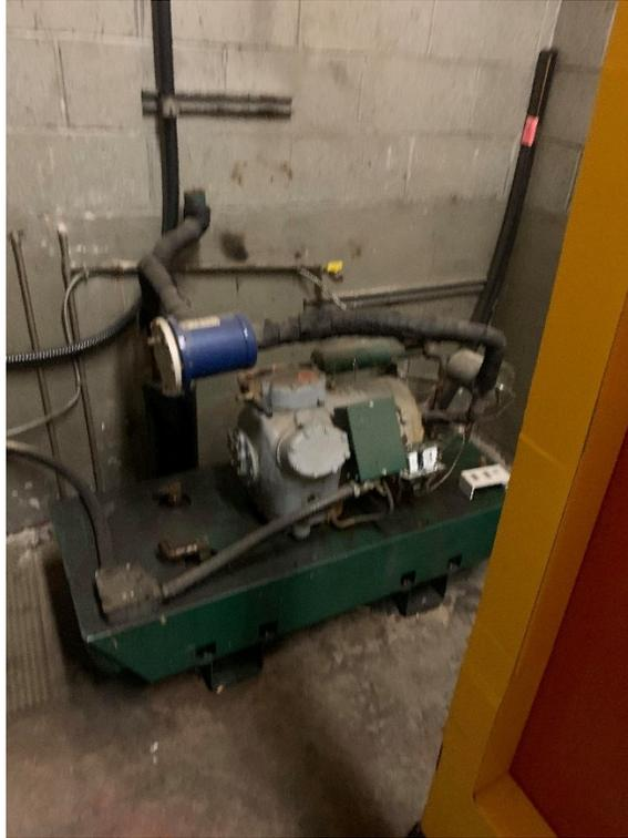
420 Lakeshore Road East: Former refrigeration unit for on-site building in mechanical room in south east corner of the building. Current refrigeration unit is natural gas and housed on the rooftop.
