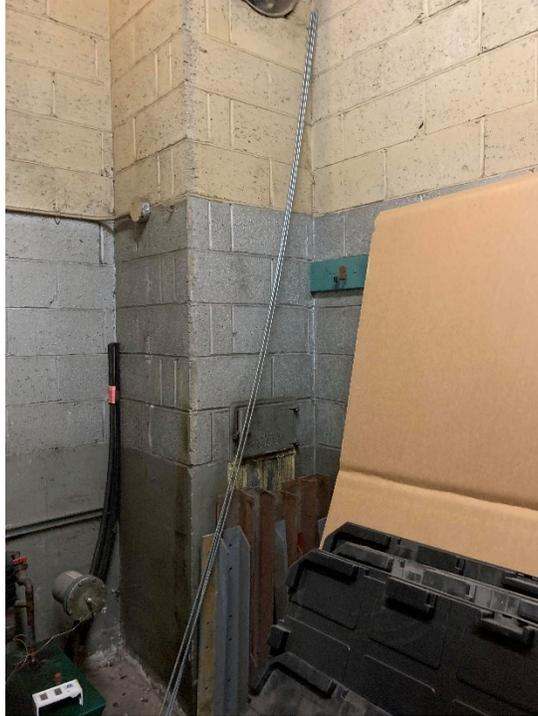
420 Lakeshore Road East: Chimney Cleanout in south east corner of on-site building. Potential evidence of historic coal usage on Site.
